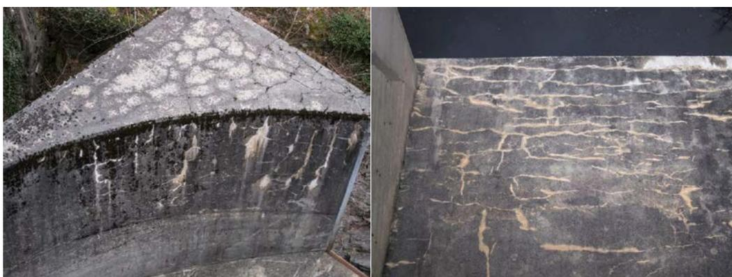
**Figure 12:** Web-shaped AAR cracks at a spillway (left) and cracks at the inlet of a spillway with prevailing crack direction due to existing forces (right).
